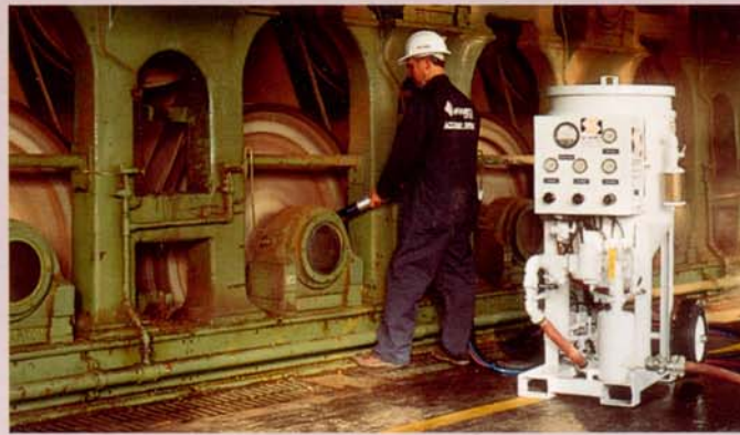
▲ Process residue quickly removed from pipes in wet end basement
