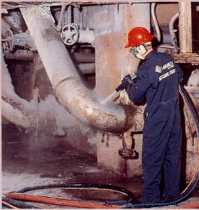
▲ Process residue quickly removed from pipes in wet end basement
